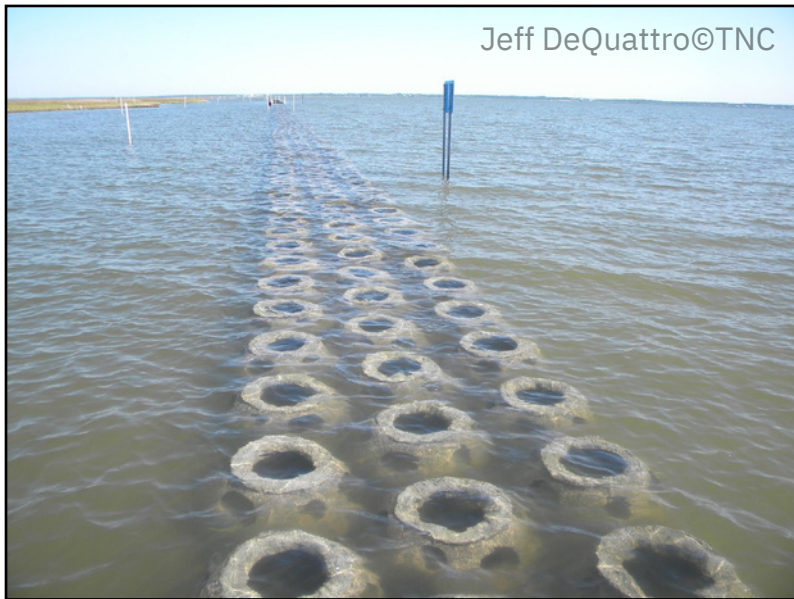
Reef Ball TM concrete domes
