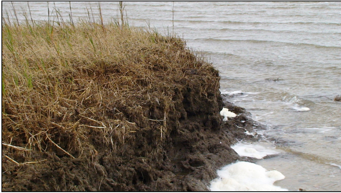
Eroded shoreline along Coffee Island, Alabama
