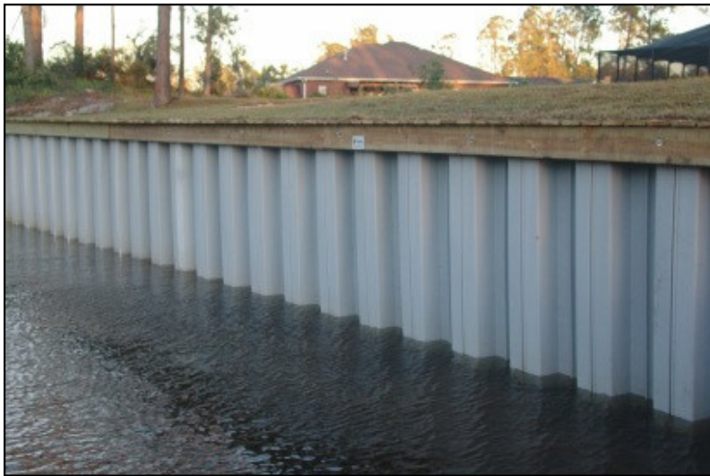
Newly installed bulkhead
