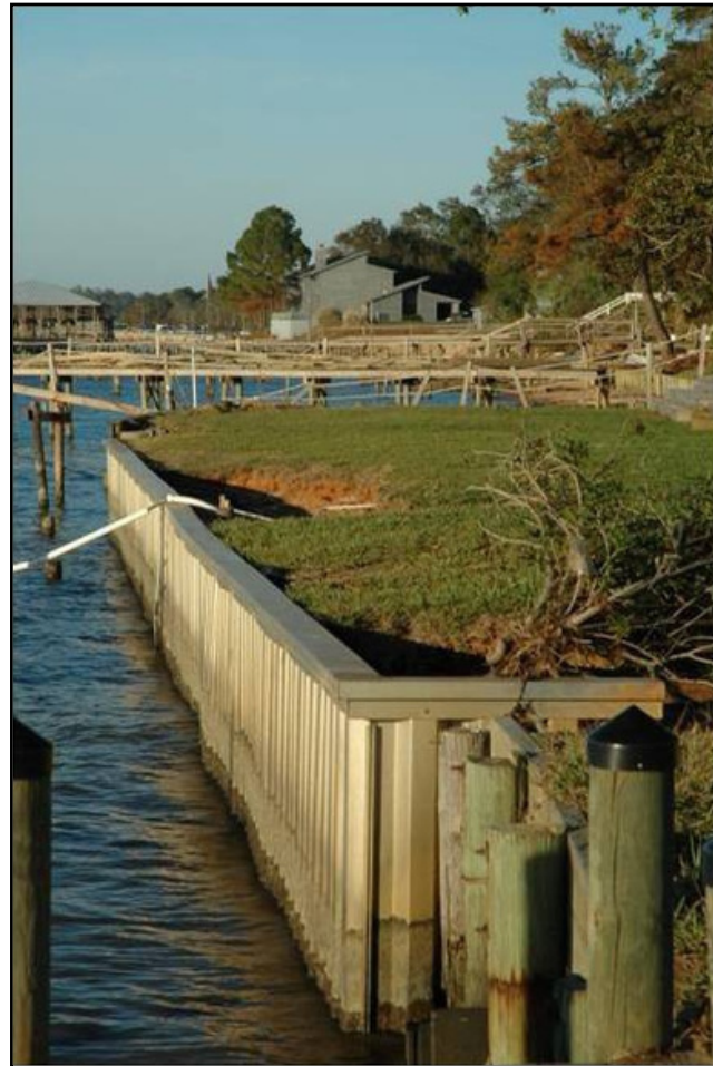
Failing bulkhead
